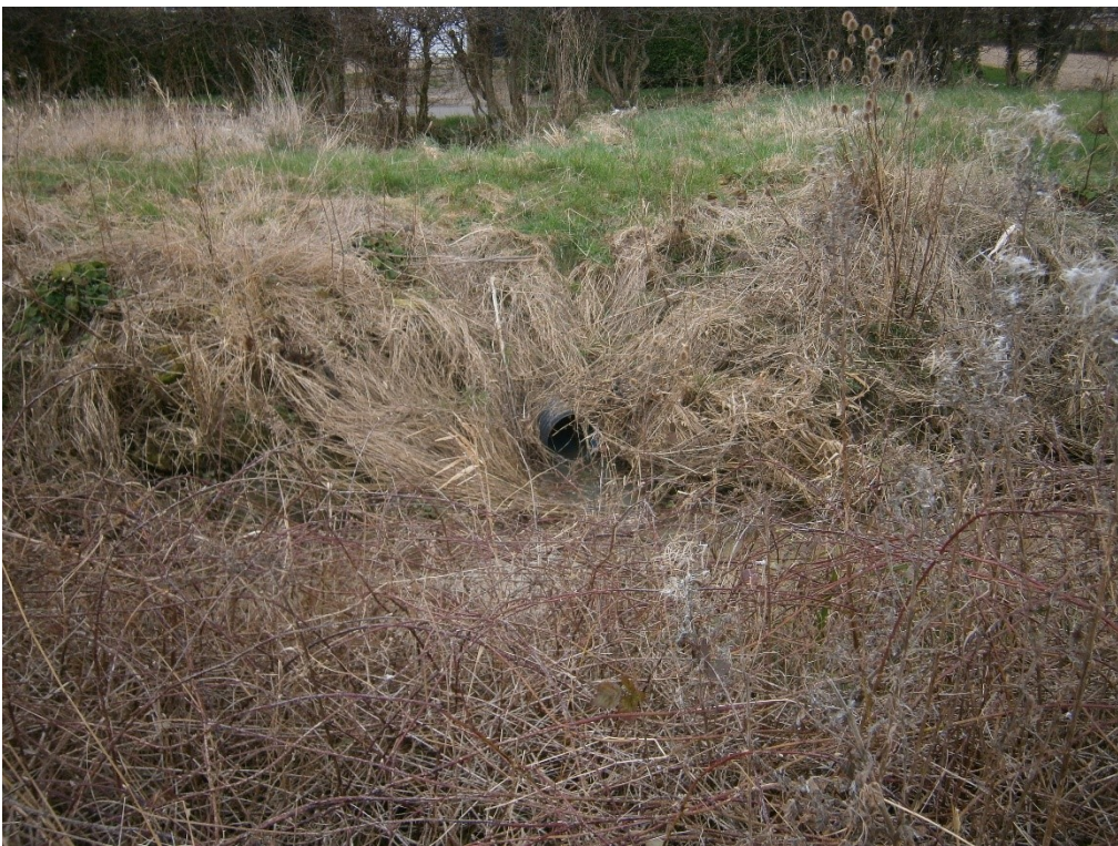
Photograph no. 10. The piped ditch on 21 February 2022.
