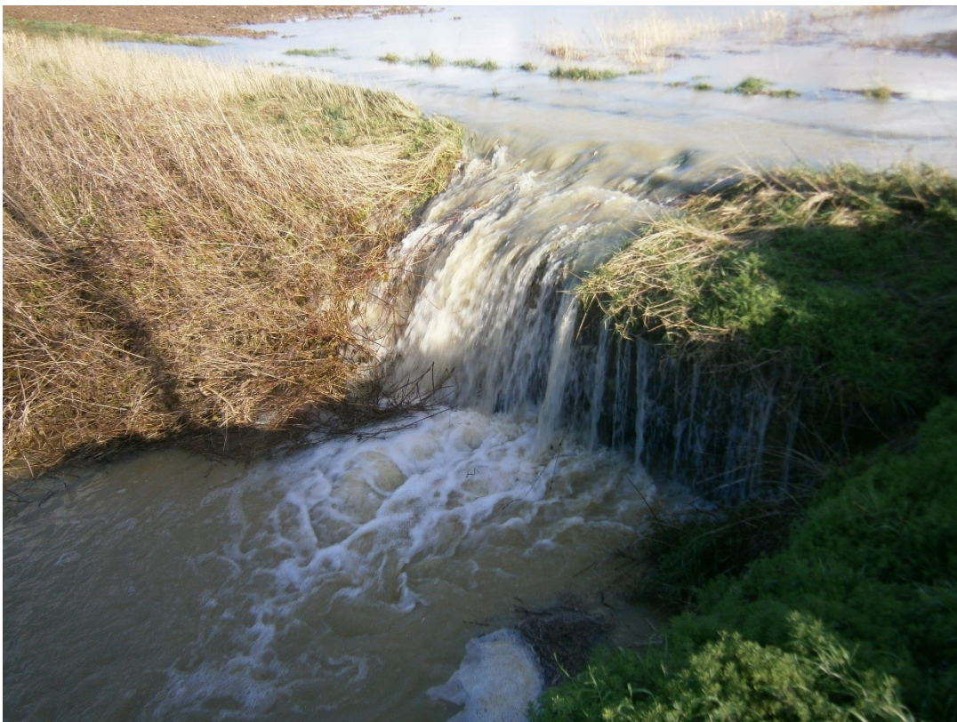
Photographs no.3 a & b taken of Restriction 2 on 29 February 2020 . Note the difference in height of the water level.
